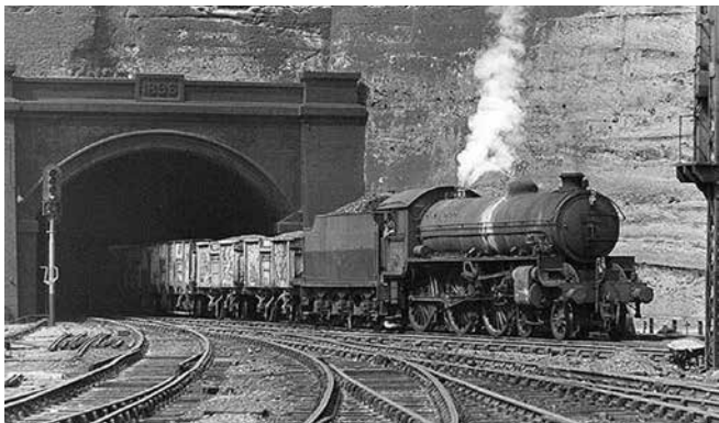
The south portal of Mansfield Road tunnel, on the north side of Victoria Station, 1962. Photo Chris Ward
